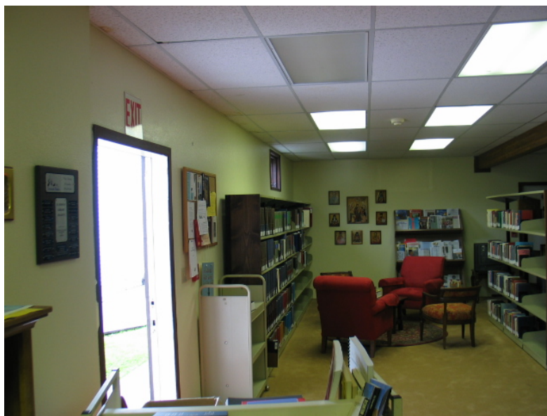
View from inside newly completed library with donor plaque placed on wall.
